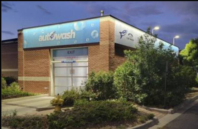
Car Wash & Other Site Buildings
